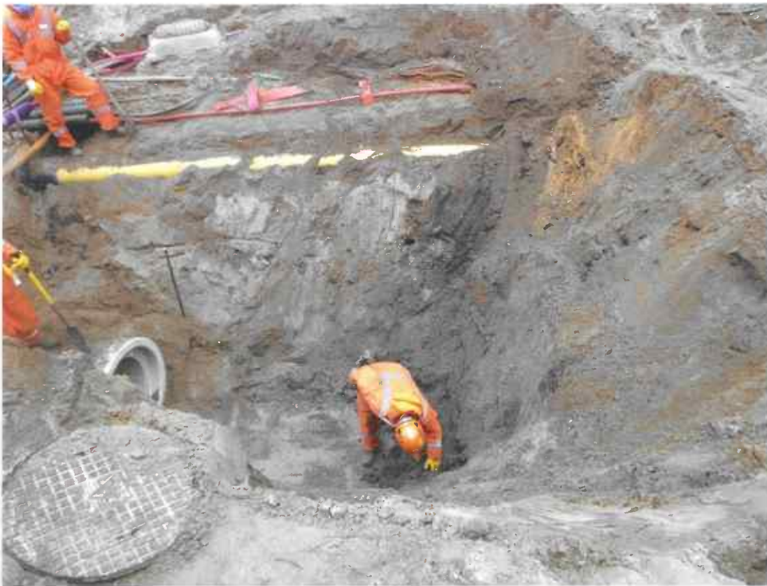
Overview of the groundwork near Stratumseind (photo: BAAC B.V.)
